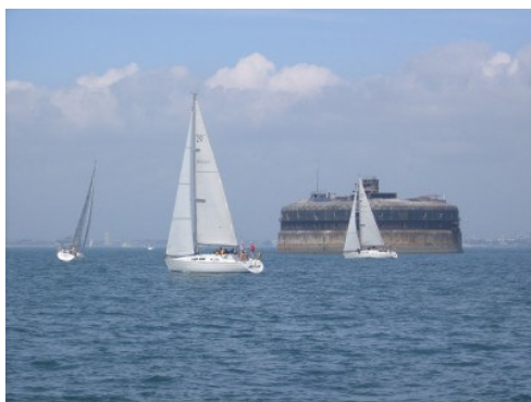
Clearing Horse Sand fort
